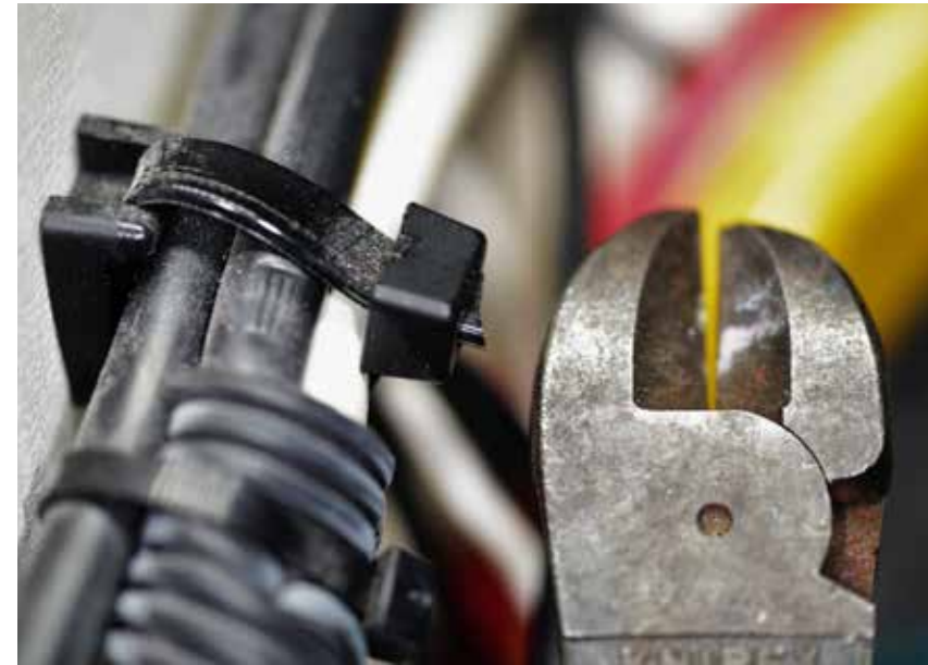
(10) The black wire tie on the left has been nipped off, leaving just enough to gash the arm of someone reaching past it.
