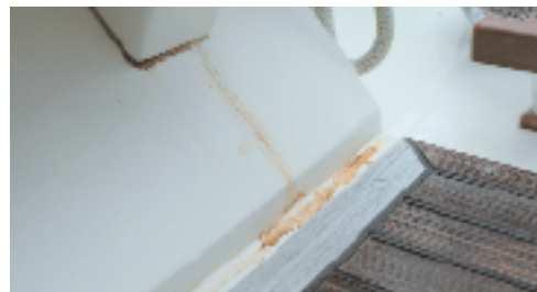
Tea-like stains are a tell-tale sign of rotting balsa core.
